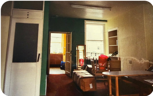
Pre Refurbishment - downstairs meeting room
