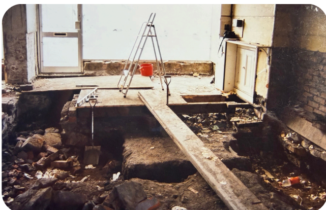
During Refurb - Reception & lift location!
