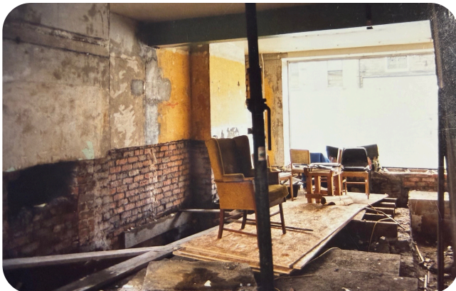
During Refurb - downstairs meeting room
